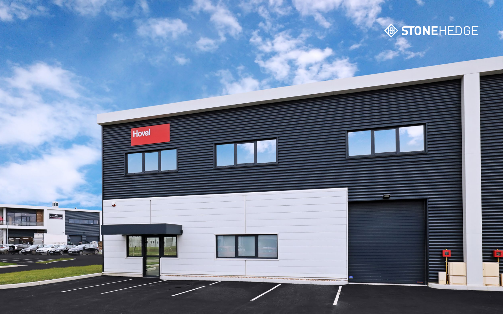
STONEHEDGE® SERVON 3 Lot A1 - Façade
