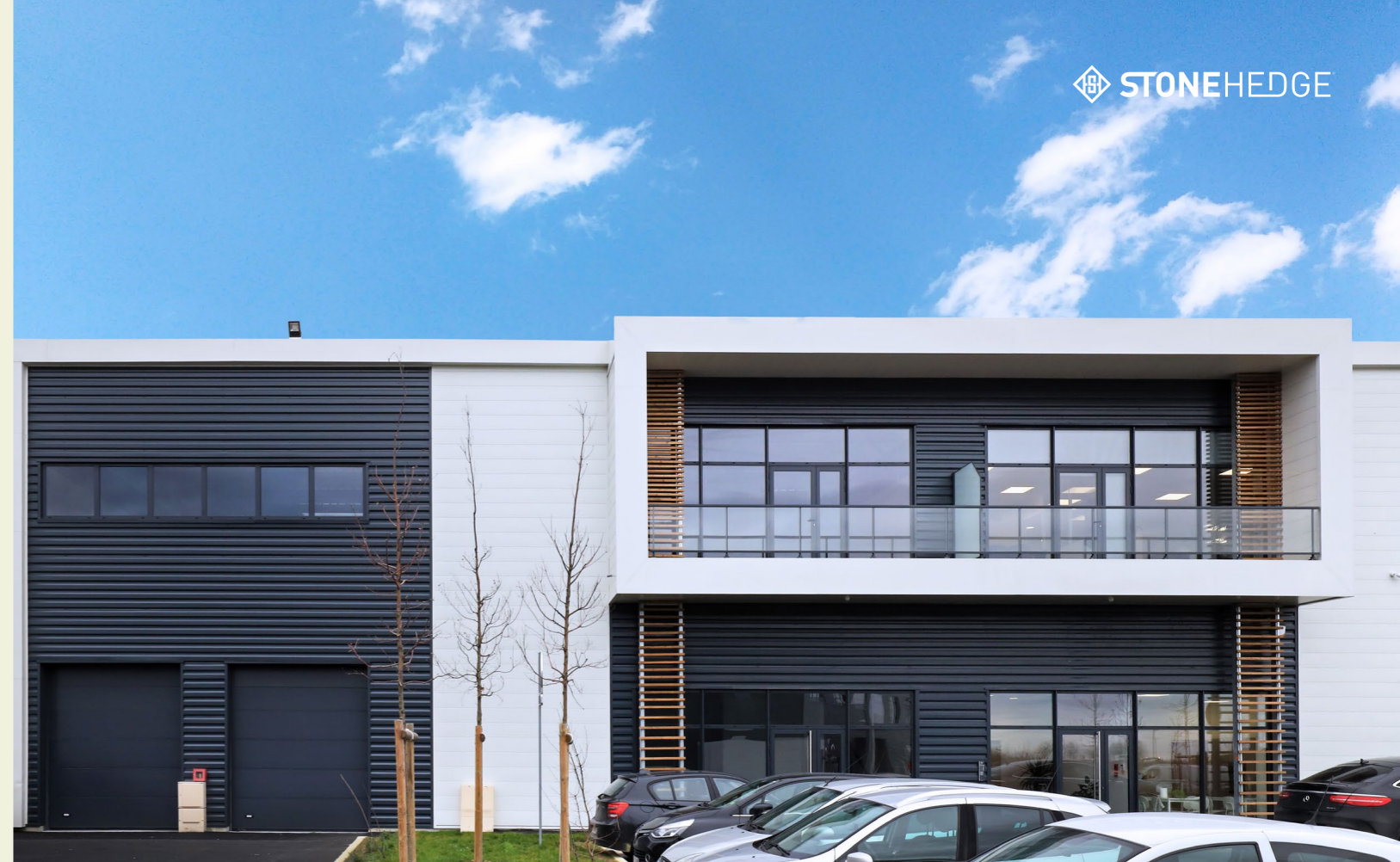
STONEHEDGE® SERVON 2 Lot E2 - Façade
